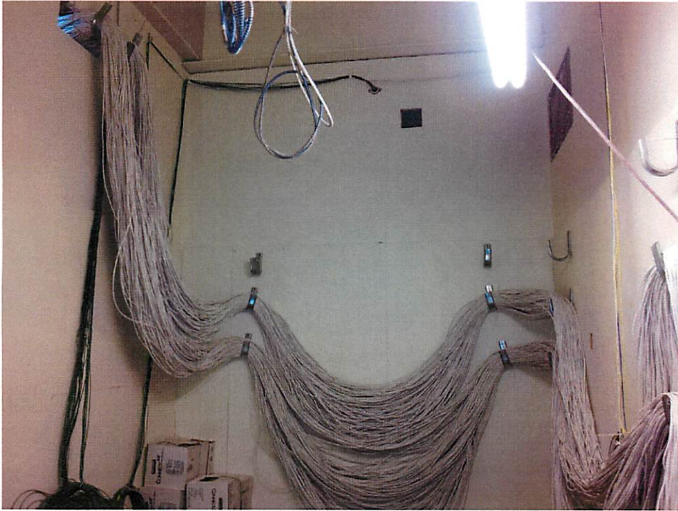
Computer Data Cable Pulls – Science Building, MDF
