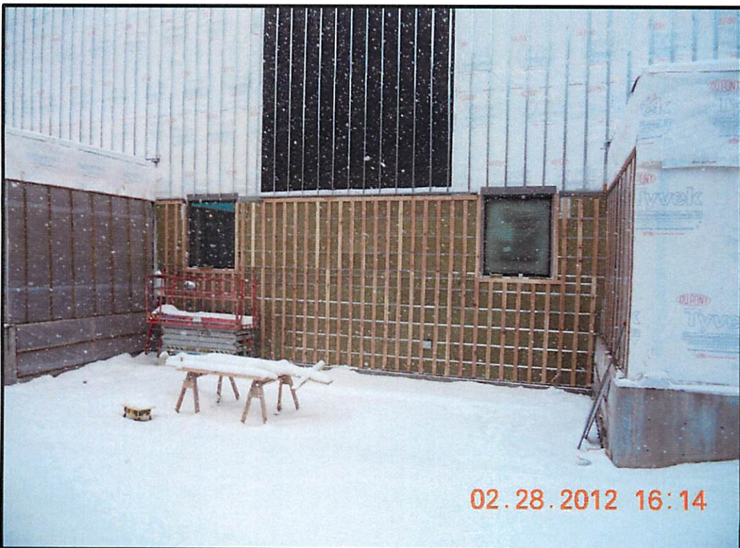
East Elevation: Substrate ready for horizontal wood siding installation.
