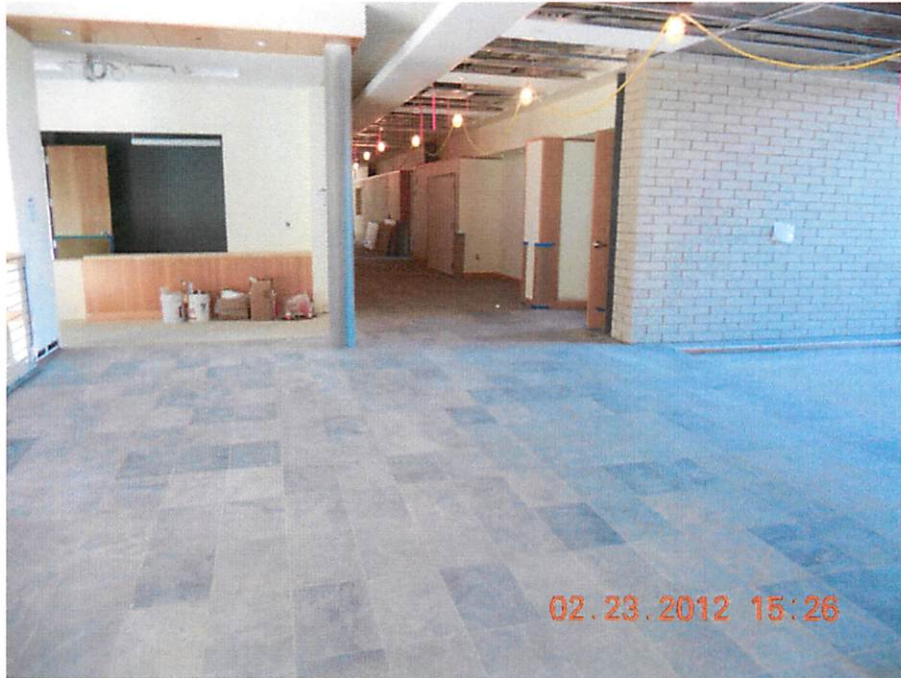
2 nd Floor looking west from top of Stair
