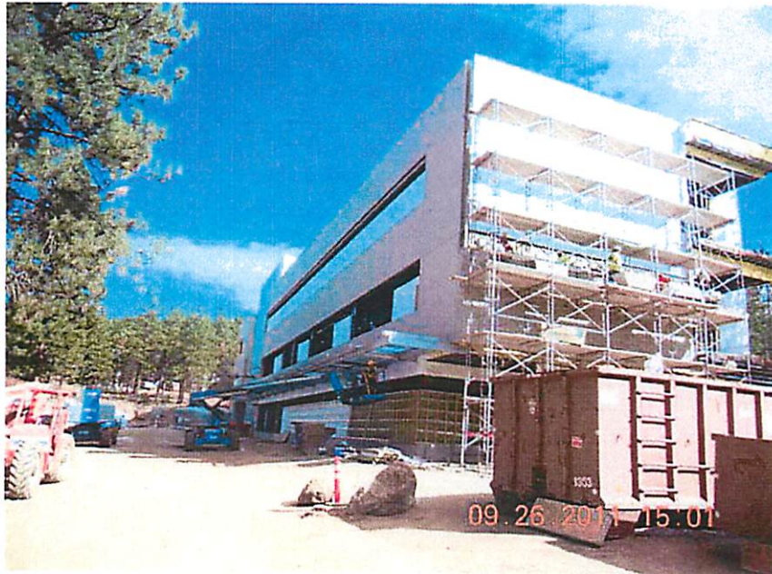
Building Wrap and Sitework
