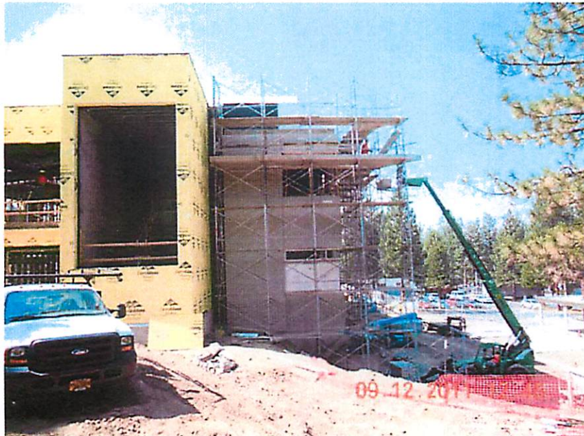
East Side Masonry
