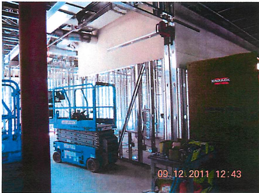
Interior Framing and MEP's Progressing
