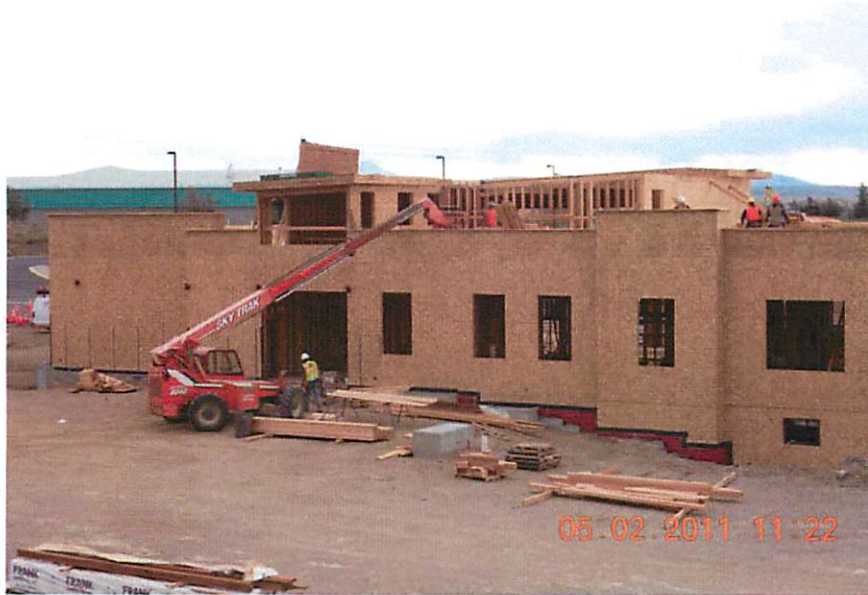
Roof sheathing and framing.
