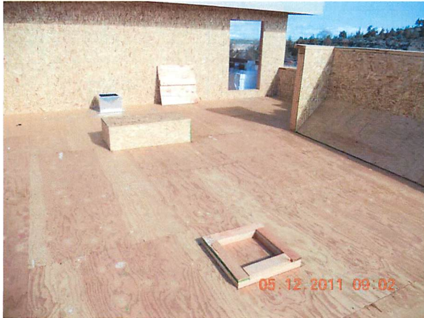
Roof just prior to roofing application.
