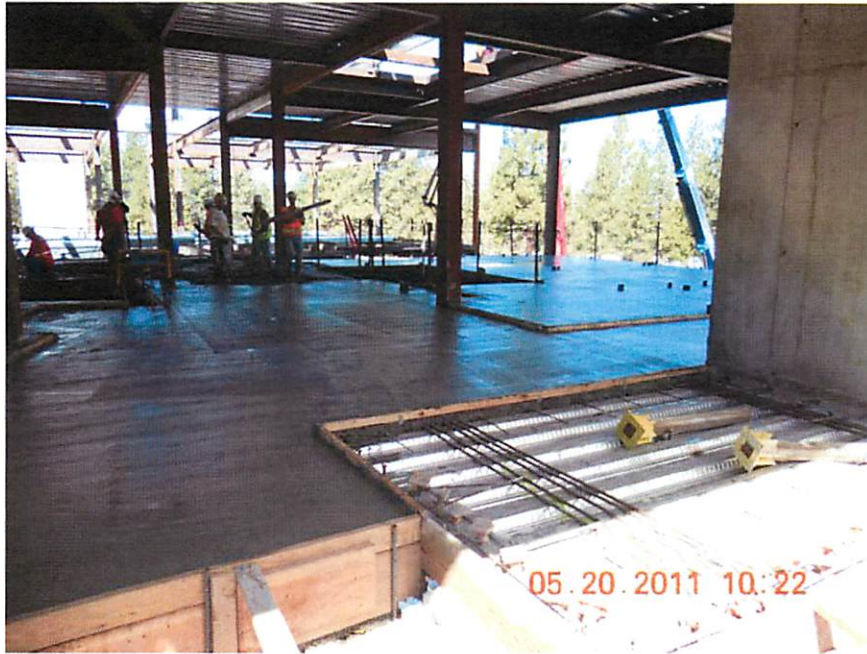
Zone 1 Floor 2 Concrete Placement
