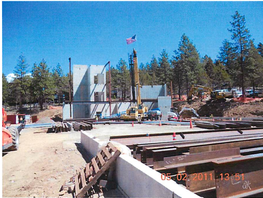
Steel Erection Commences on Zone 1
