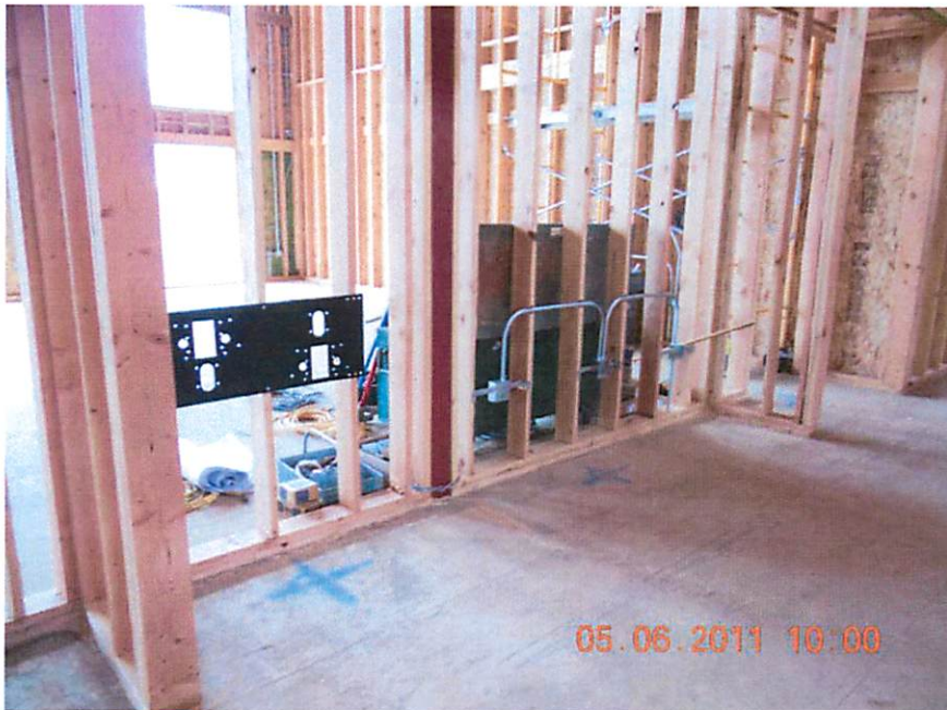
In the hall looking into the Community Room
