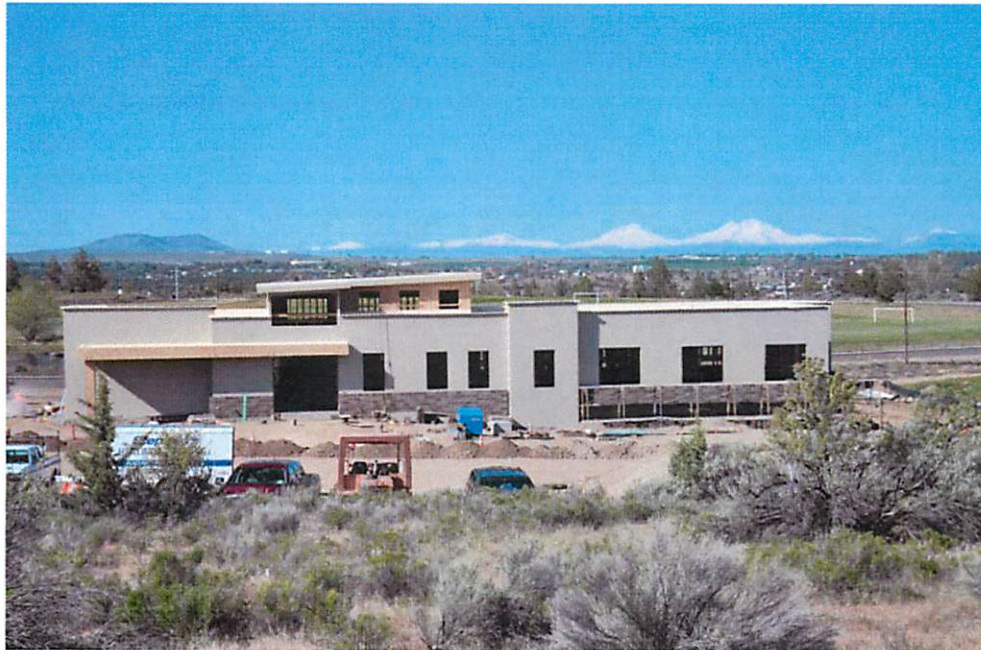
Roof complete. Lower Masonry at 80%.
