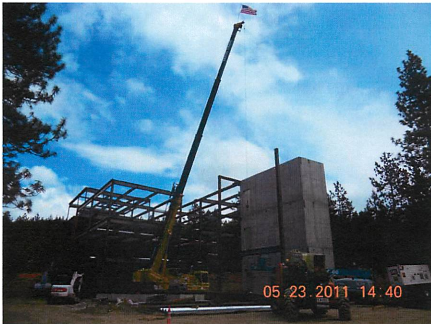
Zone 3 Steel Erection @ 50%
