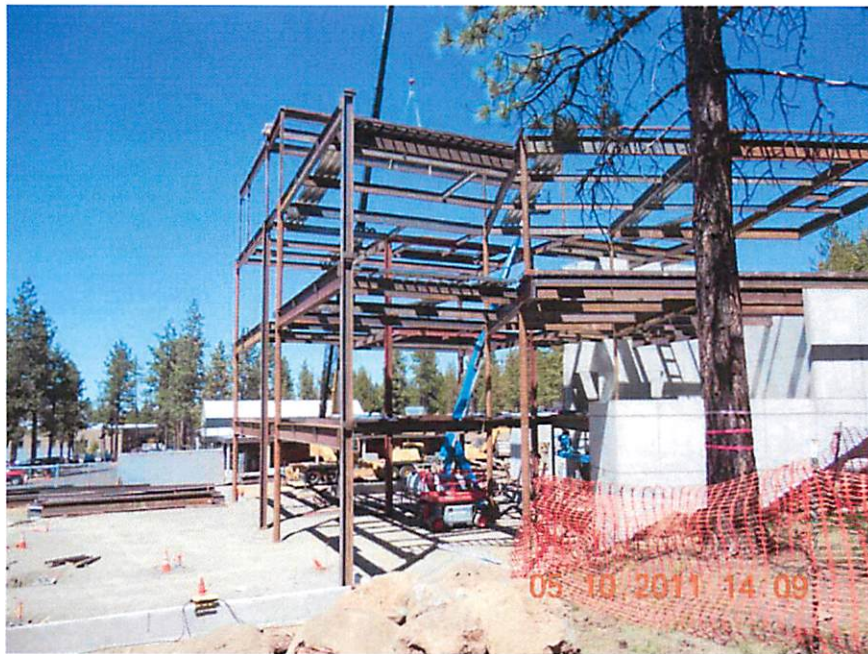
Zone 1 Complete and Ready for Decking
