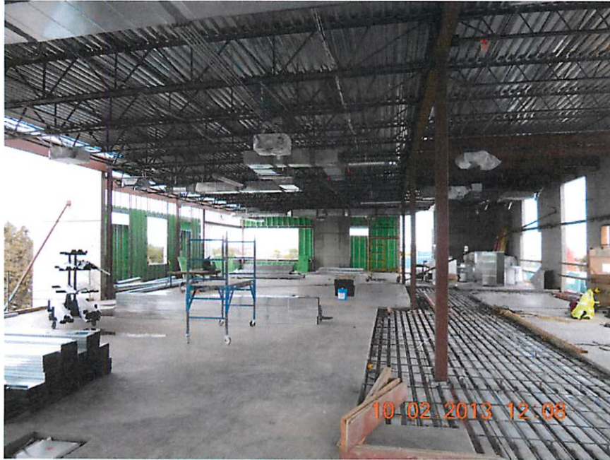
2 nd Floor South Wing Looking West
