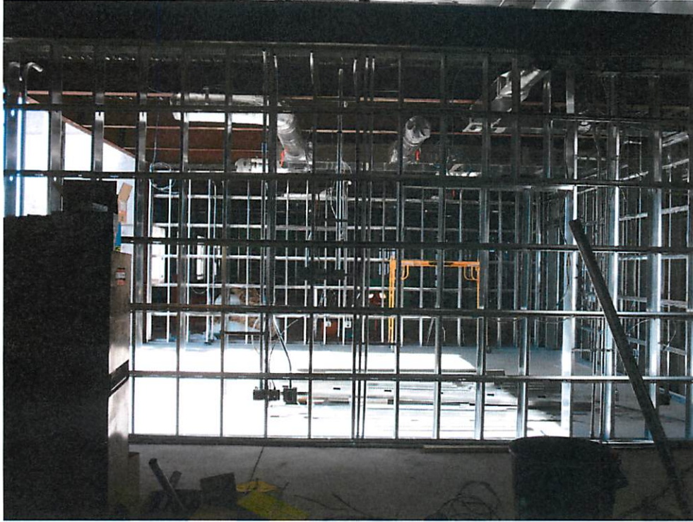
Interior Framing and Conduit Installation – South wing, Redmond Technology Center
