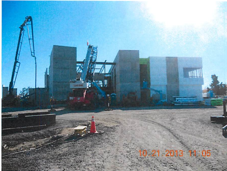
Exterior Gyp and Moisture Barrier, Roof Trusses in the Lobby
