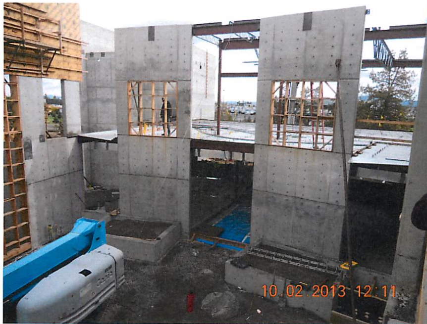
Looking into the Lobby from the 2 nd floor.
