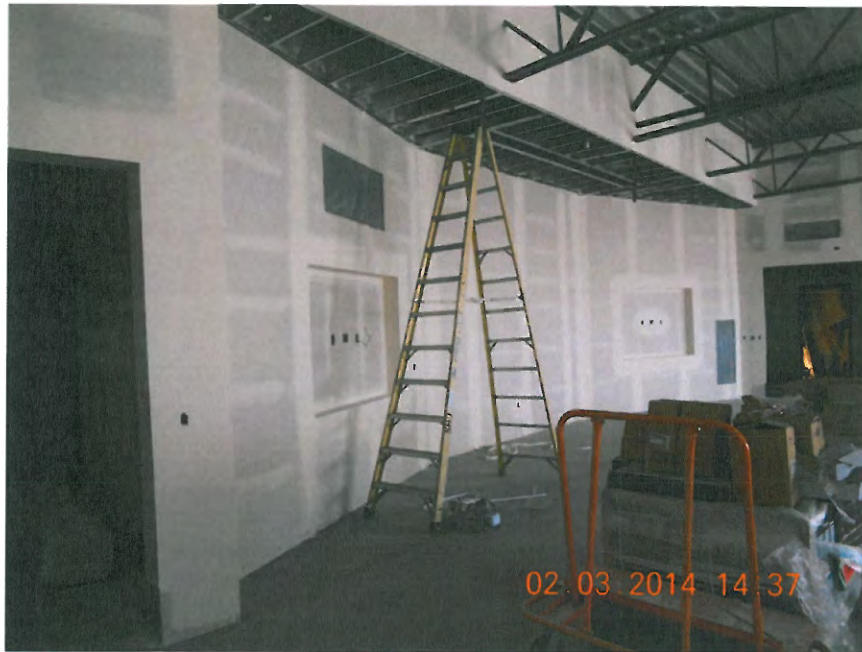
Large Upstairs Classroom
