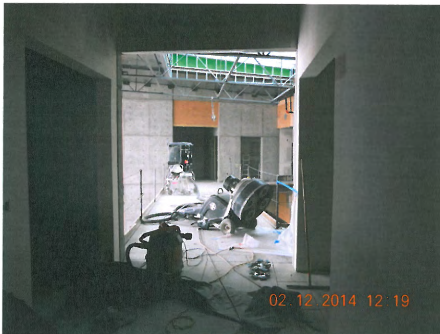
Initial Grind on Polished Floor
