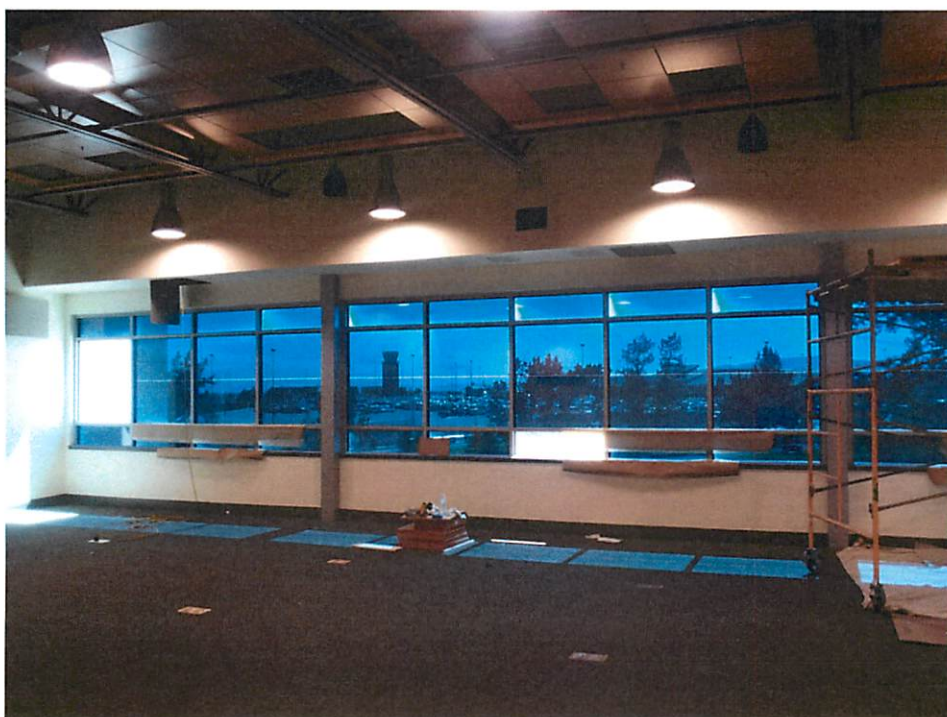
Electrochromatic glass install – Community Room 209
