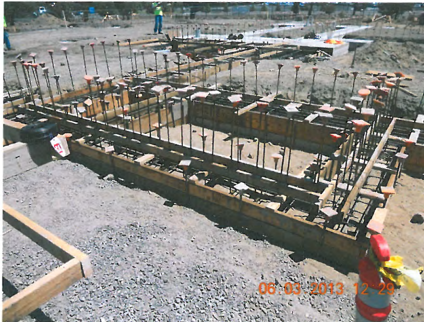
Footings at NDT/NDI X-Ray Room
