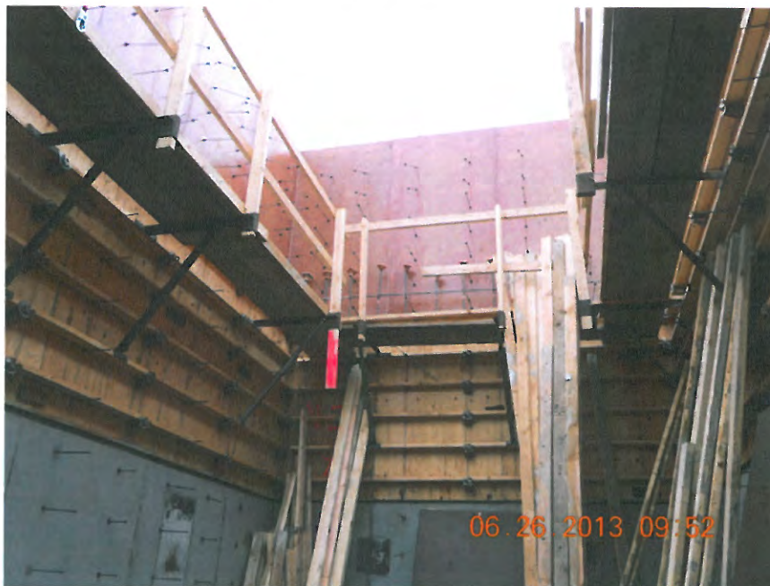
Inside Stairwell at South Wing. Forms being jumped to 2 nd lift.
