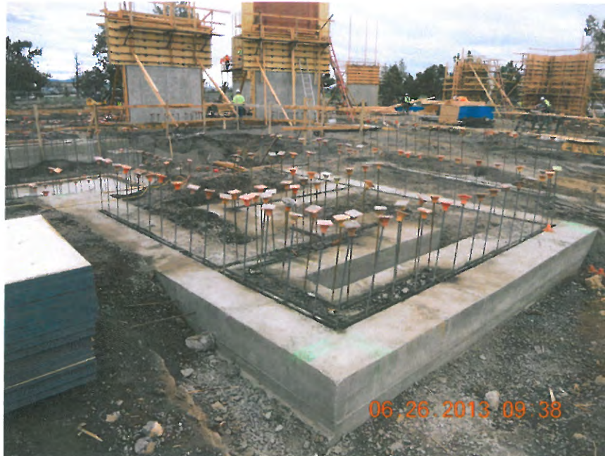
Wall forms jumped for 2 nd lift
