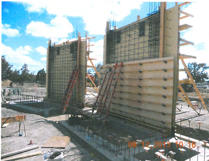
Forming Walls in Lobby behind Stairs
