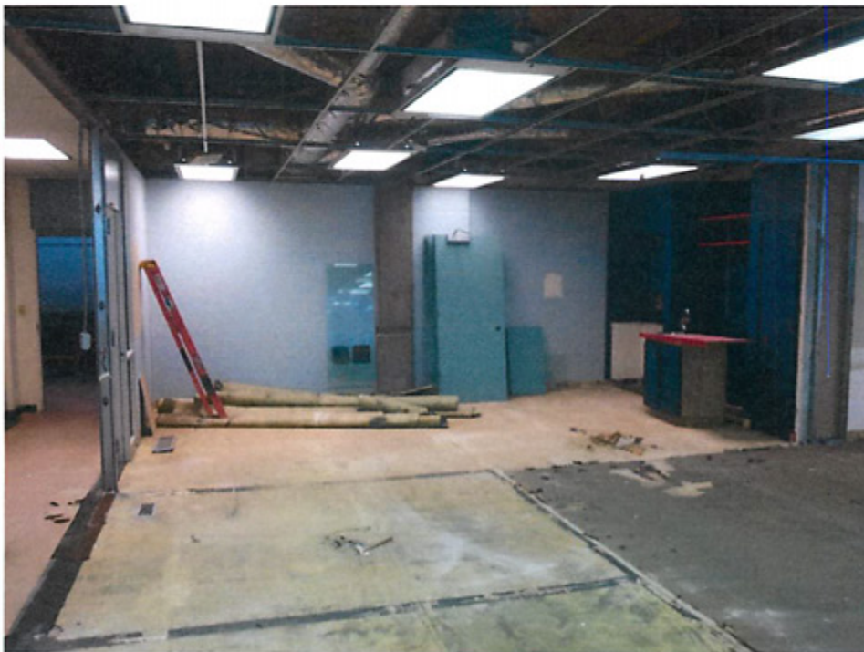
Future MDF & Computer Classroom – Pioneer remodel
